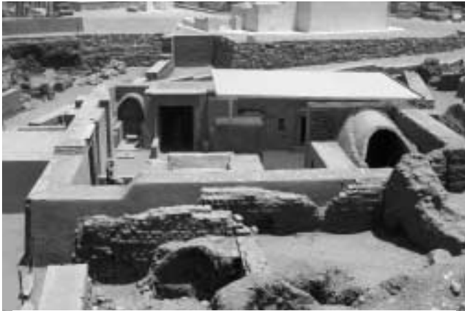
Figure 2. A simple roof structure built over a particularly important part of an archaeological site near a museum. Notice the subtle slope and gutter to direct rain away from the protected area, and avoid rising damp problems in the walls. A small price, a lot of effective preservation. All photographs in this chapter are by the author, Stefan Michalski, Canadian Conservation Institute, all except figures 9,10, made during teaching or consulting projects for UNESCO or ICOM, in or near Cairo, Aswan, and Kuwait City, between 1986 and 2002.
